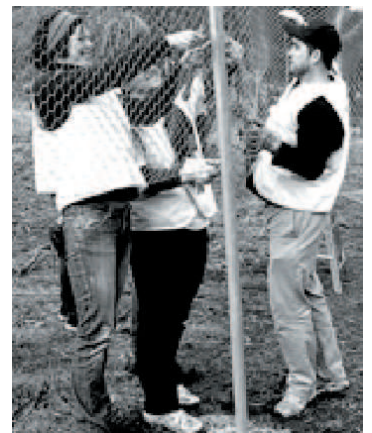
Building a fence at Woodlands Historic Park Photo: Travis Scicchitano
