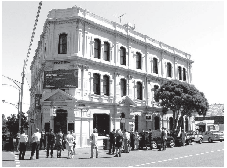
The Railway Hotel sold at auction on 23 February and is already the subject of a planning application
